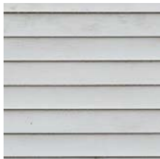
Horizontal Clapboard (existing)
